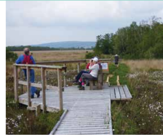
▲ New boardwalk under construction at Foulshaw Moss Nature Reserve
